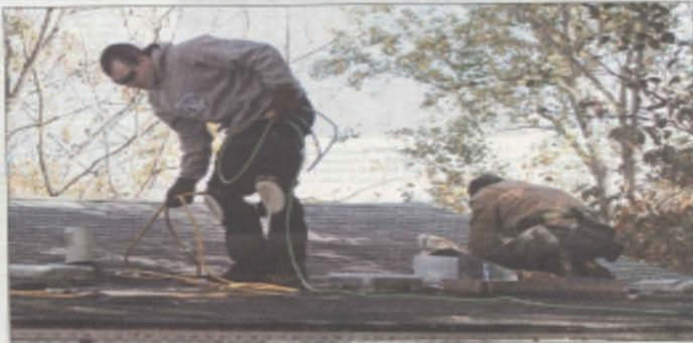
Erik Aasen, left, and Thomas Ocampo, employees of Heininger Construction of Pittsboro, inspect and replace roof sheats in the roof of Lisa Russell's home in Carrboro as part of the 10th annual Fix-a-Home event.
